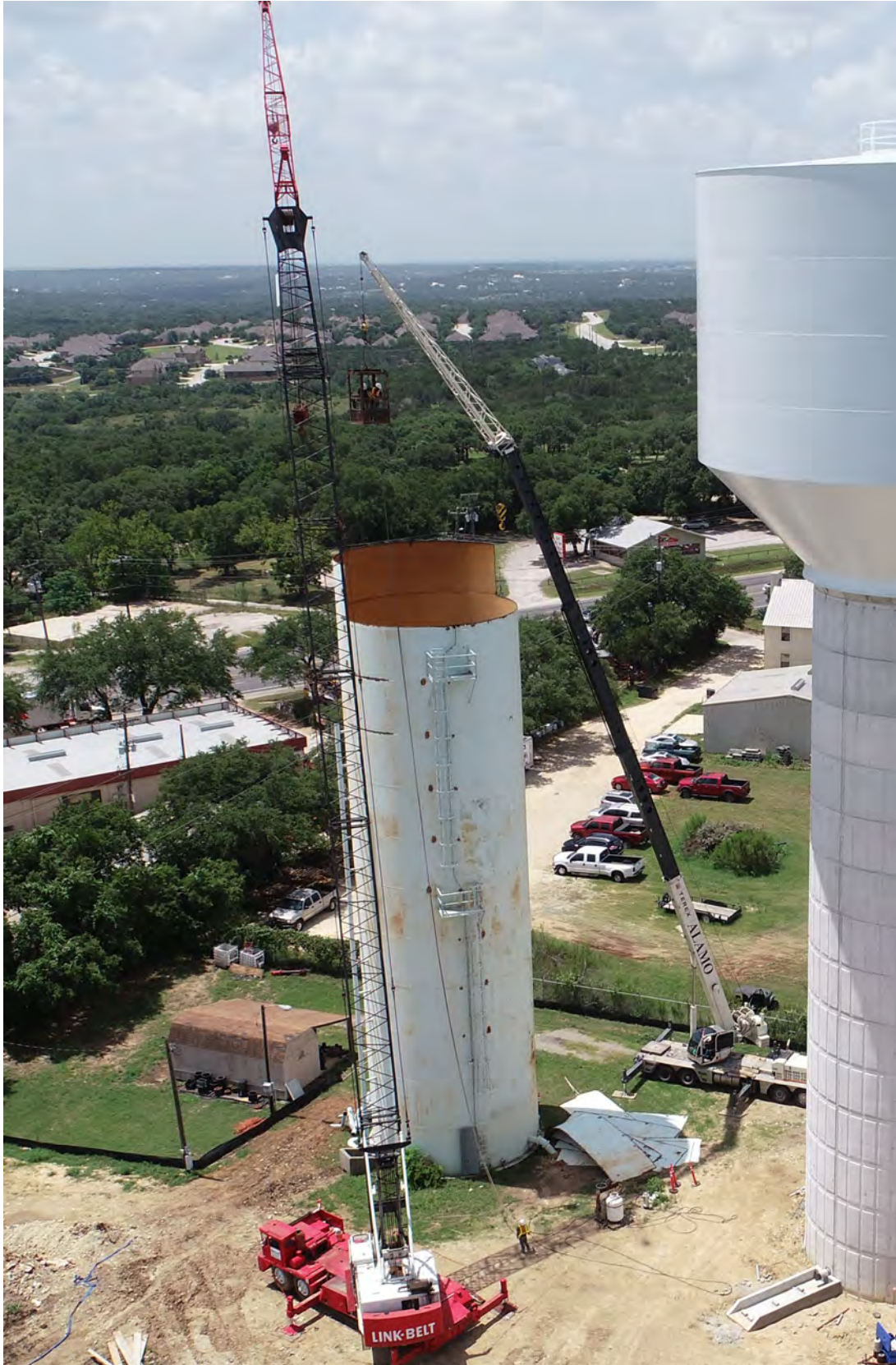
County Line 1308 Standpipe Demolition
