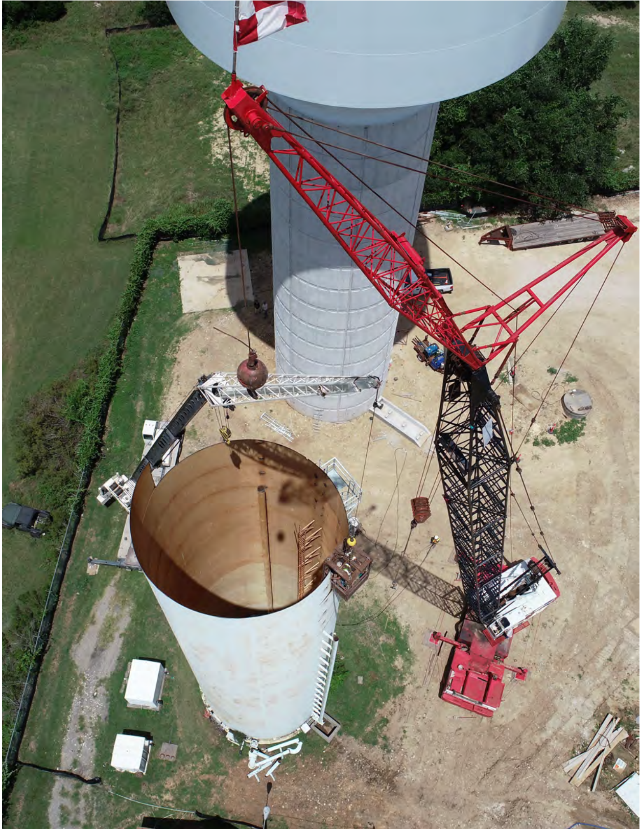
County Line 1308 Standpipe Demolition
