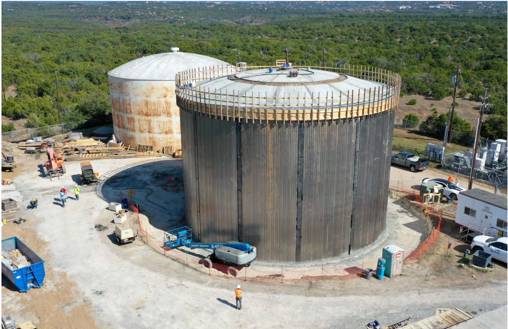
Southwest Parkway Pump Station GST 1 Foundation and Form Work
